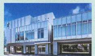
(5 Office Park, Takaoka City, Toyama)
