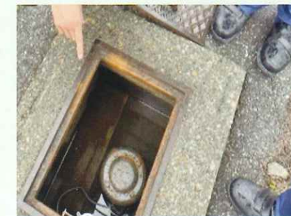
Water pipe leak detected by an IoT activity vibration sensing device
